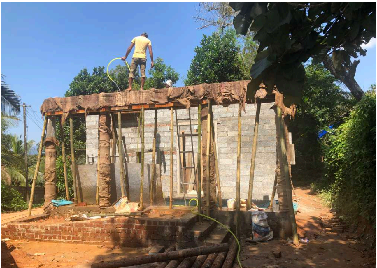
Final stages of construction at the Erumatheruv Anganwadi.
