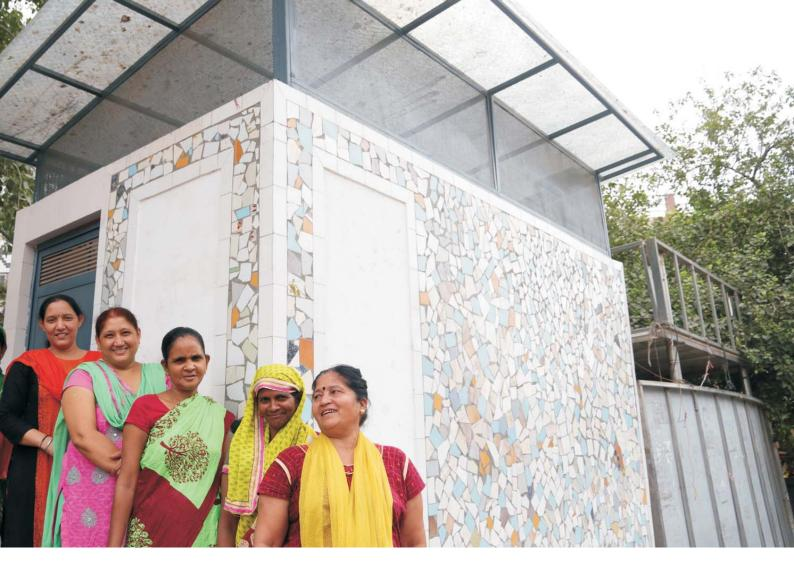
The toilet is also designed in way to support natural access to sunlight and ventilation. Solar panels ensure functionality of the toilet even during the night. Perforated jalli on all four sides ensures cross ventilations and reduction of foul smell whereas translucent fiber roof allows ambient and natural illumination by the sun during the day.
