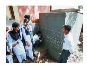
However, since rain in the area is generally limited to 2-3 months and percolation in the school premises is limited, water supply would quickly dry up. So the harvesting system was designed to ensure that it is fed by dual sources both rain and the local pond to make it functional all-year round. Rainwater pipes were installed on the roof of Block B and additional pipes connected to the pond.
