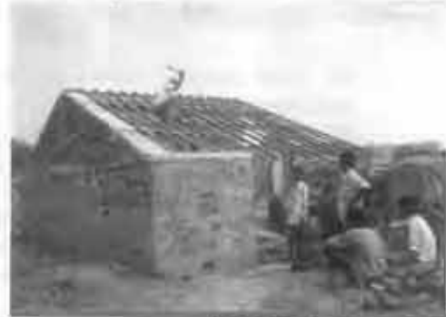
Construction of model house
