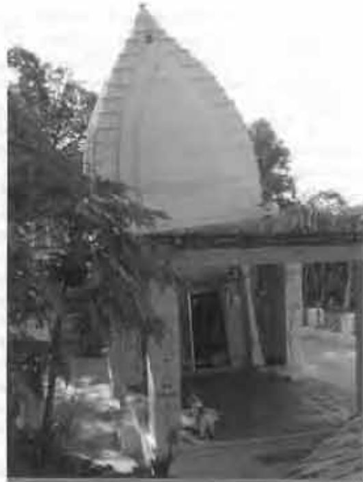
A temple affected in 1905 earthquake
