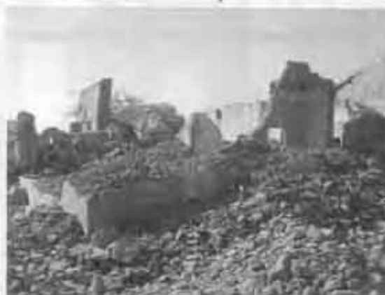
Damage in Patanka
