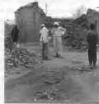
Damage in rural area
