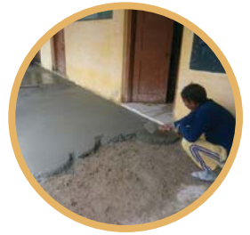
Repair of cement flooring
