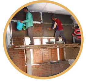
Internal wall plaster
