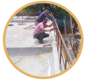
Installation of roof railing
