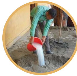
Strengthening of plinth protection
