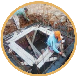
Construction of rainwater harvesting tank
