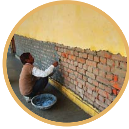
External wall plaster
