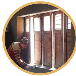
Repair of doors and windows
