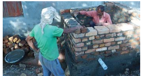
Slow sand filter under construction
