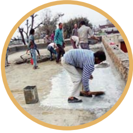
Roof cleaning, repair and waterproofing
